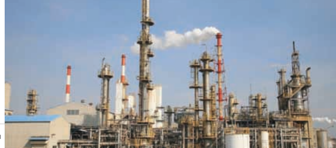
The Aboshi Plant produces acetic acid using the methanol carbonylation process.
