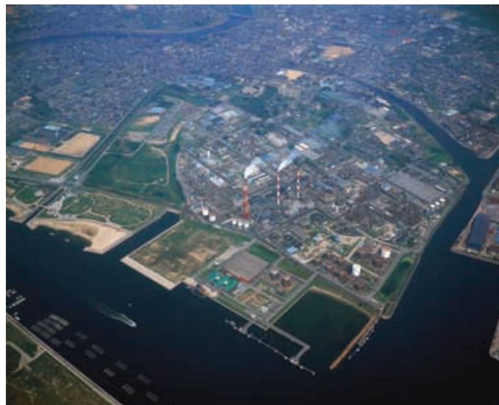
As our key plant, the Aboshi Plant (photo) manufactures cellulose acetate, acetate tow for cigarette filters, and other products from methanol, wood pulp, and other sources.
